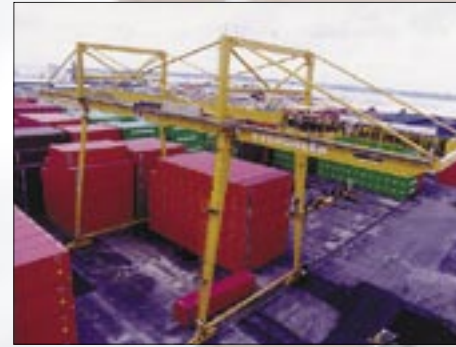
An 86m span container crane handling empty containers.
